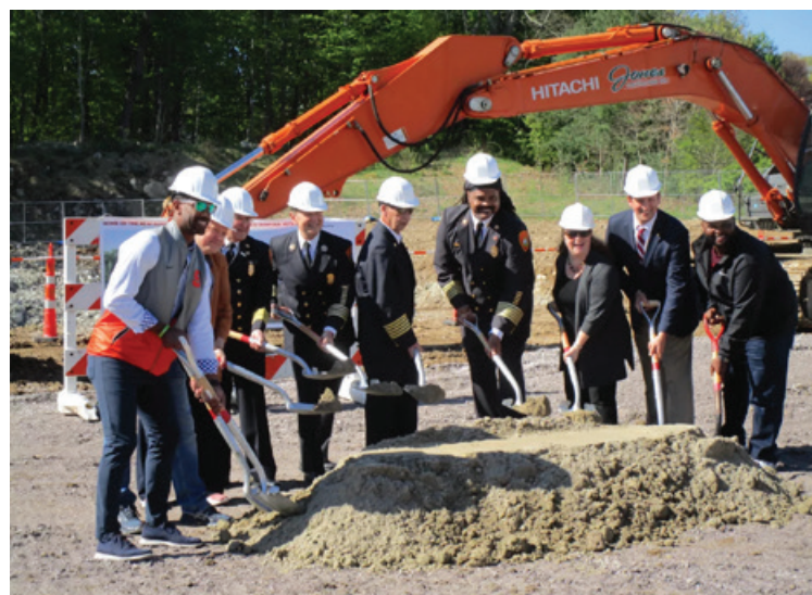
Norfolk town officials break ground at the new fire station facility site on May 6. (Photos courtesy Owner's Project Manager Steve Kirby.)
