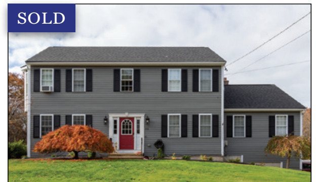
32 Field Pond Road, Milford
