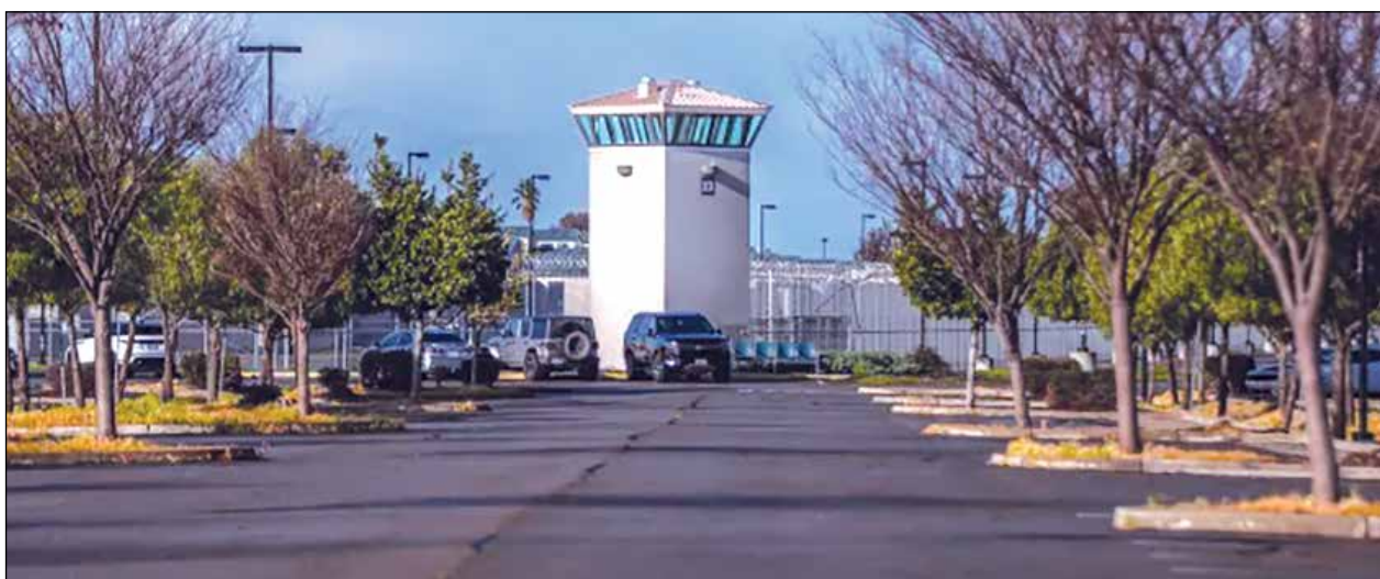
A watchtower at the California Health Care Facility in Stockton on Feb. 5, 2023. Photo by Rahul Lal, CalMatters
