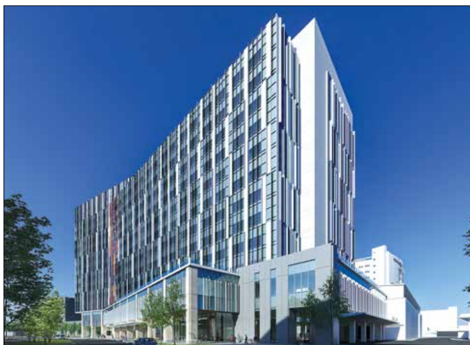
The California Tower adds to the Medical Center's existing University and Davis Towers and will add approximately one million square feet of additional space. Photo courtesy of UC Davis Health
