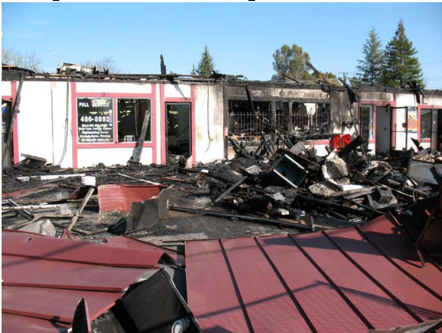
Early Morning Blaze Destroys Businesses
