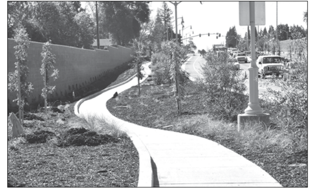
The county's Department of Transportation received an award for the Hazel Avenue Improvement Project which widened the road from 4 to 6 lanes to reduce congestion from Highway 50 to Madison Avenue. Photo courtesy of Sacramento County
