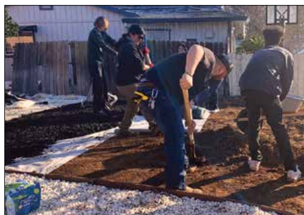
Workers from a dozen Home Depot locations donated their time, skills and expertise to this Rebuilding Together Sacramento project. Photo courtesy of the City of Rancho Cordova
