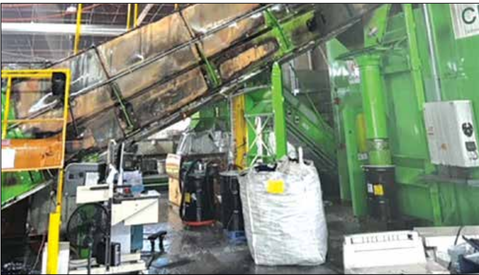
A fire in the very large e-waste recycling warehouse in Mather presented a challenge to Sac Metro Fire units due to interior smoke and a faulty hydrant. Photos courtesy of Sac Metro Fire
