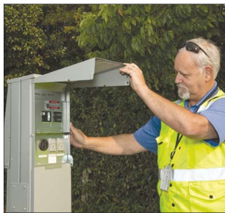
Sacramento Municipal Utility District (SMUD) Program Manager David Hatfield inspects newly installed "shore power" electric hookups at the Sacramento 49er Travel Plaza, a truck stop near the interchange of Interstates 80 and 5. By providing utility power where big-rig drivers spend their rest periods, truckers can plug in their rigs to electrical outlets and avoid idling their engines. By doing so, truckers save money and harmful emissions are reduced.
