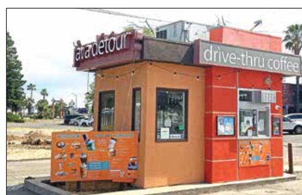
The closed 106-square-foot Java Detour coffee kiosk is expected to be demolished. Photo by Thomas J. Sullivan
