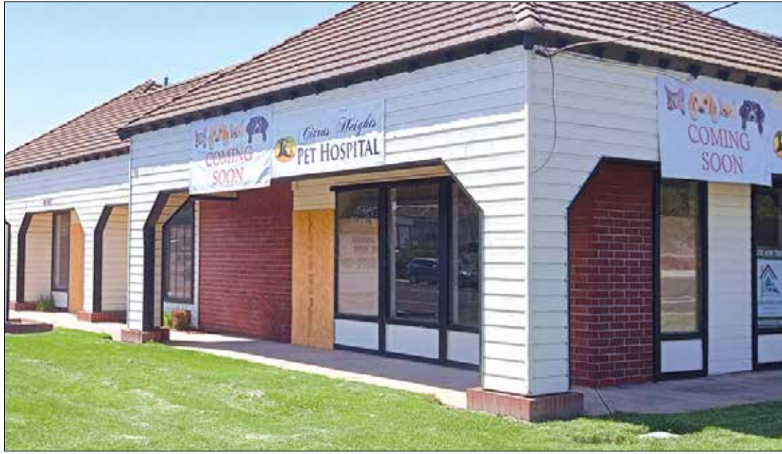
Citrus Heights Pet Hospital, founded in 1962, will be moving in August to its new location in the Greenfaire Village Center.
