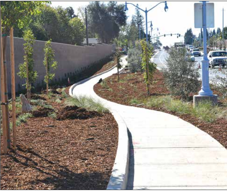
The county's Department of Transportation received an award for the Hazel Avenue Improvement Project which widened the road from 4 to 6 lanes to reduce congestion from Highway 50 to Madison Avenue. Photo courtesy of Sacramento County
