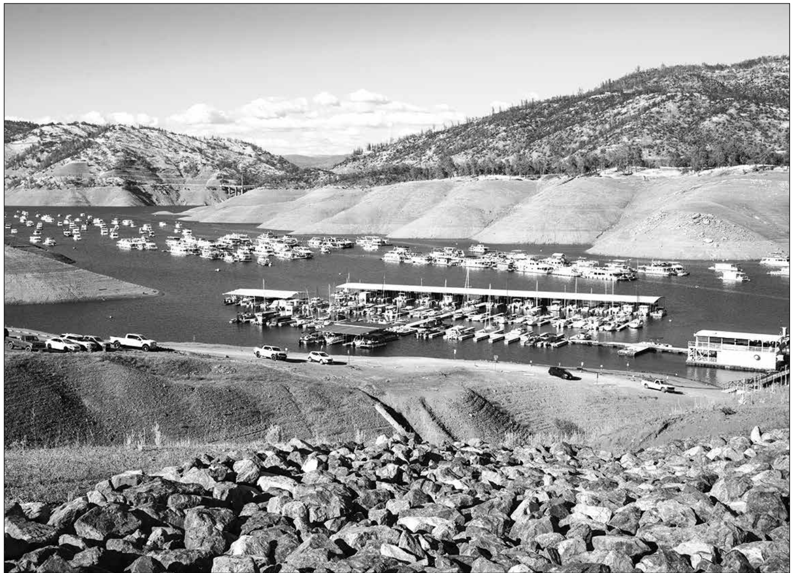
Bidwell Canyon Marina showing Lake Oroville with a reservoir storage of 1,663,134 acre-feet (AF), 47 percent of the total capacity. Lake Oroville is located in Butte County, California. Photo taken July 6, 2022, by Florence Low/California Department of Water Resources
