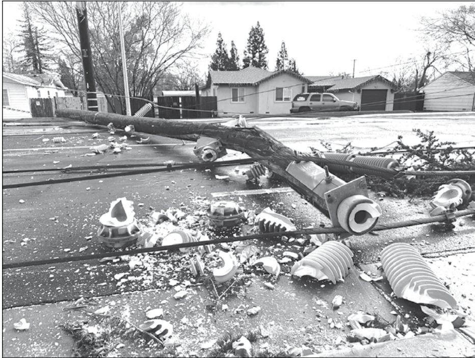
SMUD crews were out in full force to repair damage caused by the high winds. Photo courtesy SMUD.
