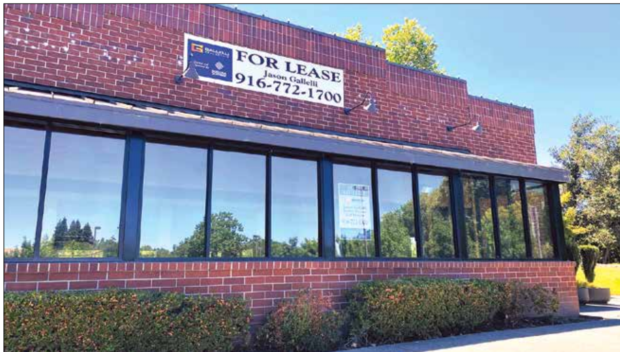
The site of the closed Applebee's would make a great place for an Aisle 1 gas station. Photo by David Dickstein
