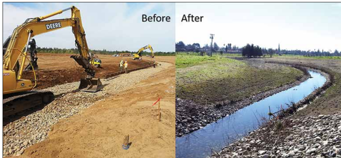
Cordova Creek Naturalization Project during construction and after.
