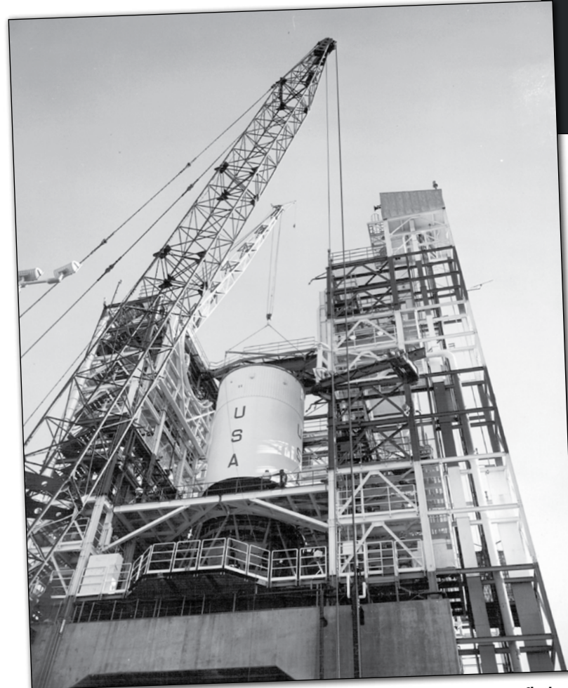
Once the stage arrived at the test site, the stage was lifted from the flatbed truck and onto the test stand. The Douglas Aircraft Company tested the third stage of the rocket known as S-IVB at its test site, the Douglas Aircraft Sacramento Test Facility in what is now Rancho. Testing of the S-IVB began in 1963 and was a significant component of the Saturn V Rocket in the future moon missions. Photo courtesy of Center for Sacramento History, Douglas Aircraft Company/NASA Employee Collection, 2014/015.
