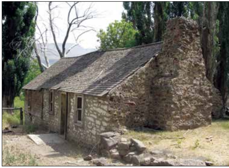
Camp McGarry Mess Hall – still standing today at Soldier Meadows, this rock-constructed building was used in the mid-1860's as a dining facility for the outpost U.
