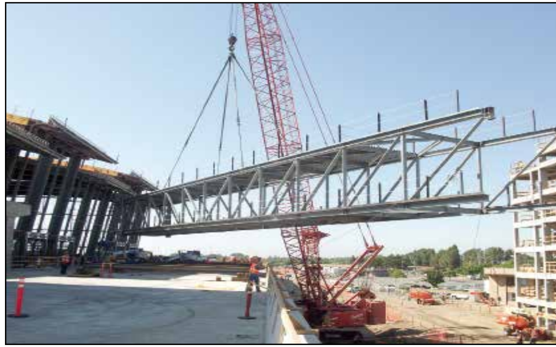
The first of three terminal bridge sections is now in place.
