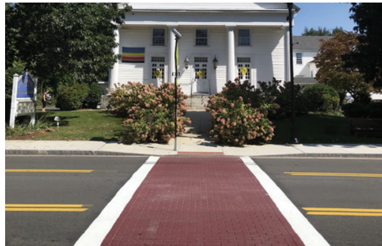
Ashland streetscape work is expected to be completed in Oct. as part of the downtown revitalization project. Improvements included sidewalks and crosswalks that are actually stamped asphalt.
