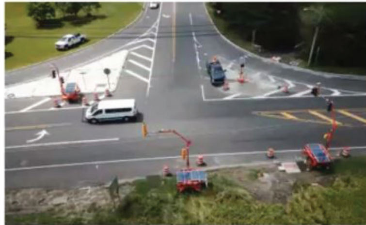
Photograph 10: Temporary Traffic Signals (Trailer Mounted)
