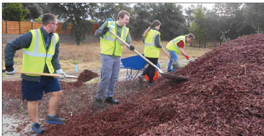
Yellow vested volunteers spread about fifty piles of rich brown bark with rakes and shovels.
