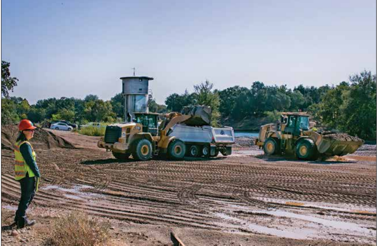
Carmichael's iconic water tower stands amid the $3.6 million project to restore salmon spawning beds on the American River. Water Forum Habitat manager Erica Bishop watches excavation progress near Ancil Hoffman Park.
