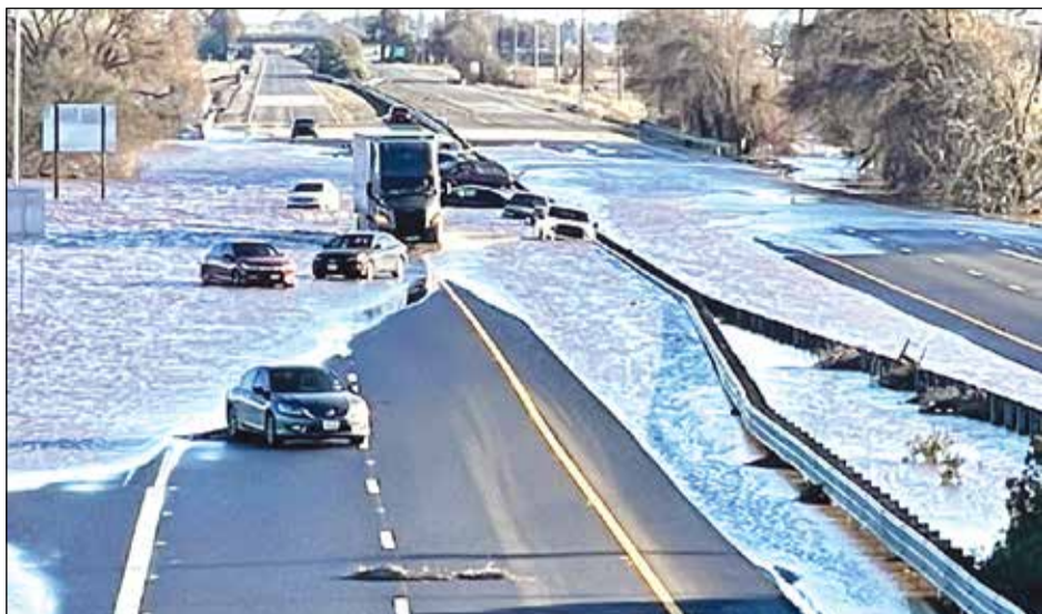
Flooding on Highway 99 at Dillard overpass last winter. Photo courtesy Sacramento County
