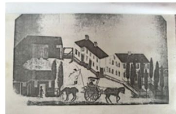
From an 1814 tax assessor drawing, historians know the Center School lot once was the site of the David Fisher Dry Goods store, left, and the Roebuck Tavern, right, among other buildings. Dedham St. is in the foreground. Wrentham Historical Commission.
