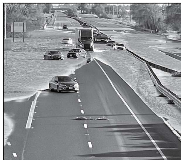
Flooding on Highway 99 at Dillard overpass last winter. MPG Courtesy Photo
