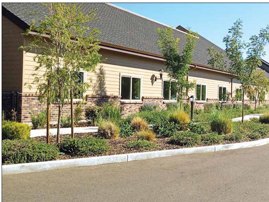
The 40,000-plus-square-foot facility, called Shadowbrook Gardens, sits on 3.72 acres at 5915 Dewey Dr. in Fair Oaks.
