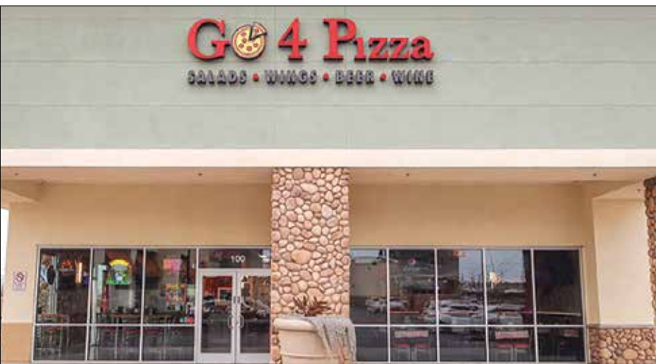
The outside view of Go 4 Pizza's Rancho Cordova location. Photo provided by David Nguyen
