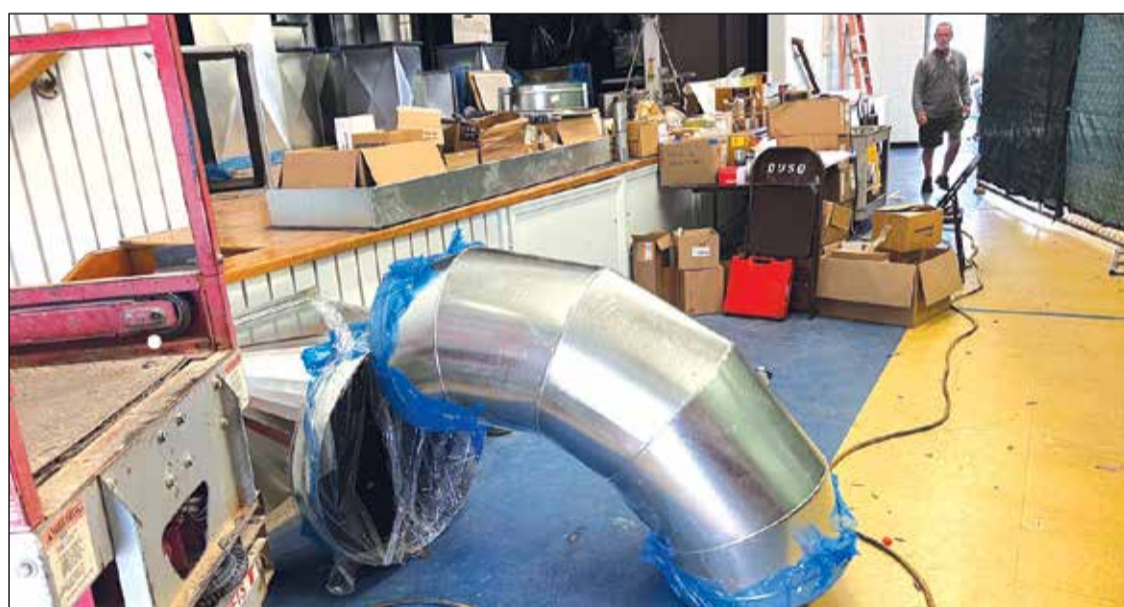
Construction supplies fill much of the multi-purpose room.
