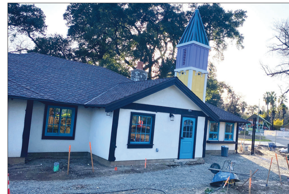
The new welcome center is almost complete.
