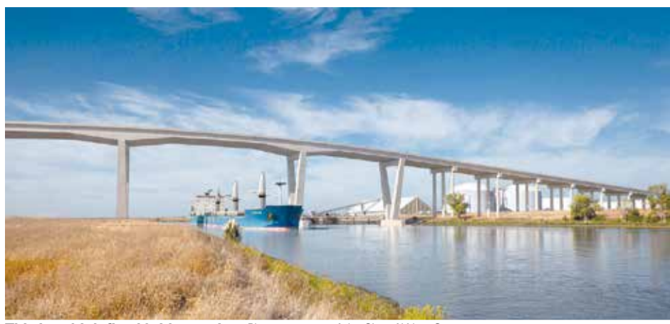
This is a high fixed bridge option. Photo courtesy of the City of West Sacramento
