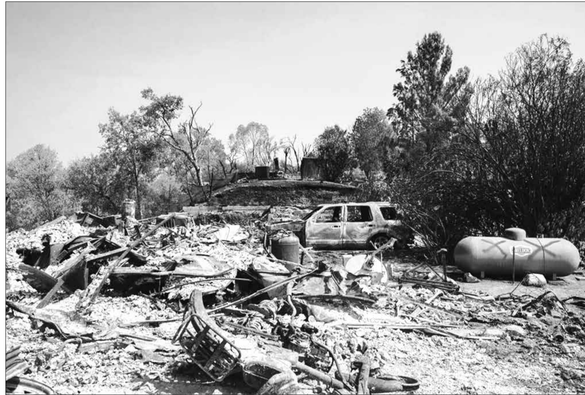
Here are the remains of a burned home in Berryessa Highlands on Sept. 21, 2020. Photo by Anne Wernikoff for CalMatters
