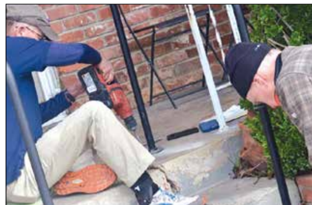
Safe at Home volunteers Dan Ward, of Carmichael, and Stan Jones, of the Greenhaven/Pocket area, install a handrail for a Sacramento resident in need of safer step way. Photo courtesy of SAFE Credit Union
