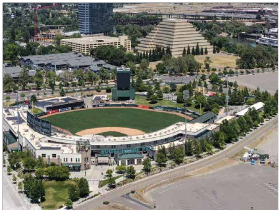
Here is the Sutter Health Park entrance, which will welcome thousands of Oakland A's fans now that the Major League Baseball team will call West Sacramento home temporarily. Photo courtesy of West Sacramento
