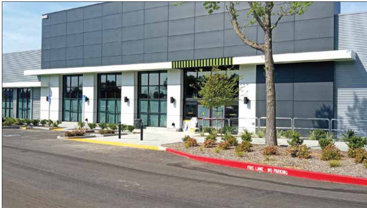
The grocery store set to occupy this space has not been named publicly yet.
