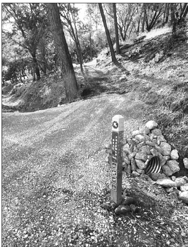
Trailhead marks the start of rerouted trail. Photo courtesy of California Department of Water Resources
