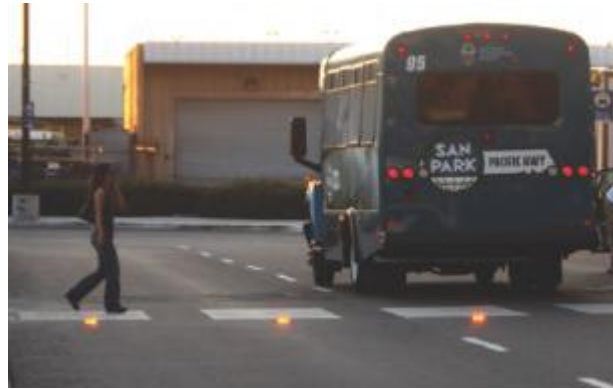
Pavement lights in crossing
