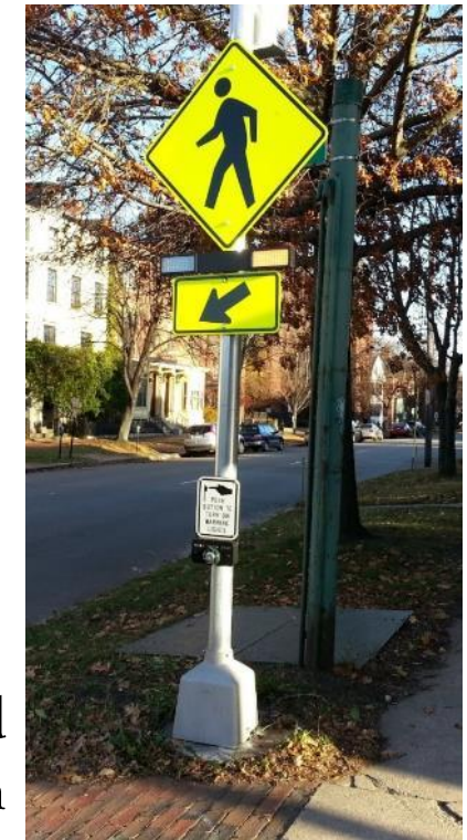
Pedestrian Rapid Flashing Beacon
