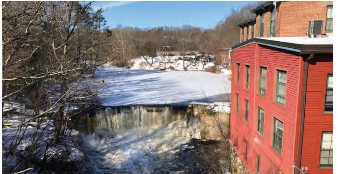
A view of the waterfall at Sanford Mill Condos after a heavy snowstorm in late January was followed by freezing rain in early February. Credit Theresa Knapp
