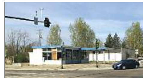
The controversial 'Old Chevron Station' at Eagle Road and State Street.
