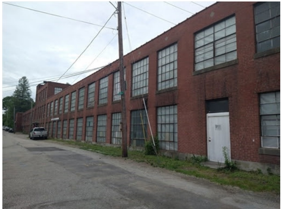
The former Anglo Fabrics buildings in Webster are soon to become the focus on a major redevelopment project.
