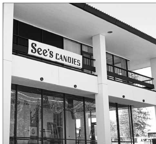
The See's store at 5499 Sunrise Boulevard now showcases the recently repainted black and white See's company colors.
