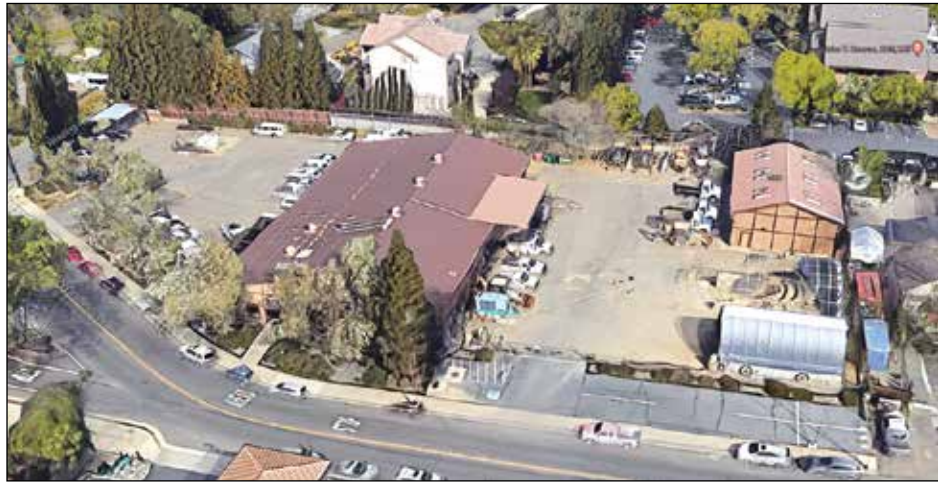
Aerial view of the FOWD Corporation Yard located at 10317 Fair Oaks Blvd in Fair Oaks, Calif. Photo courtesy of FOWD
