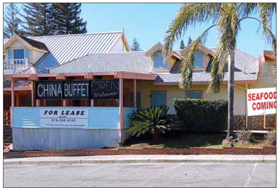
Outdoor signage announcing the pending opening of a seafood restaurant on the site has since been removed by the owner/broker Jarrett Real Estate of El Dorado Hills, which continues to market the property as an active listing. Photo by Thomas J. Sullivan
