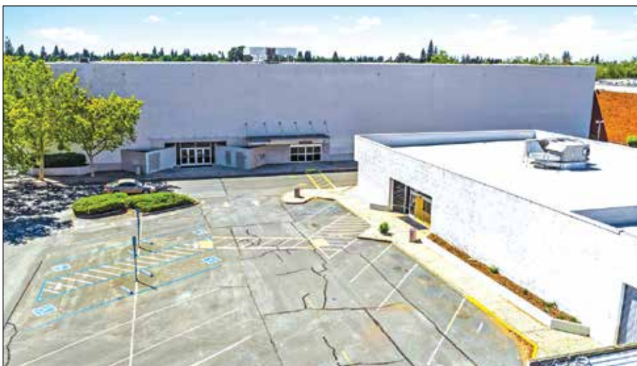
Colliers Retail Capital Markets image of Sunrise Mall Sears building now listed for sale for $8 million. Photo courtesy of Sunrise MarketPlace
