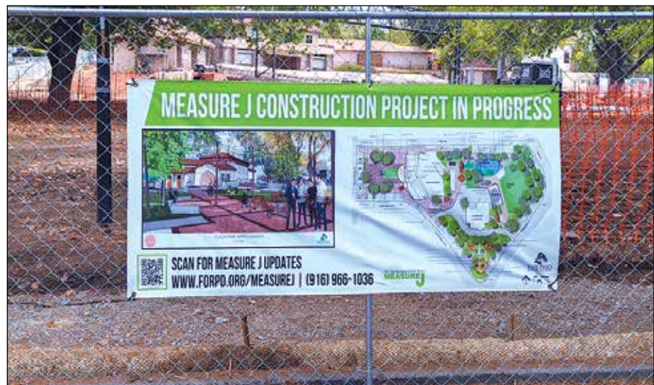
Construction in the Village is currently underway, and the $21.7 million project will include improvements to Plaza and Village parks, updates to the Community Clubhouse, and a new theater building at Veterans Memorial Amphitheatre. Work is expected to be completed in December 2023. Photo by Shauna Boyd
