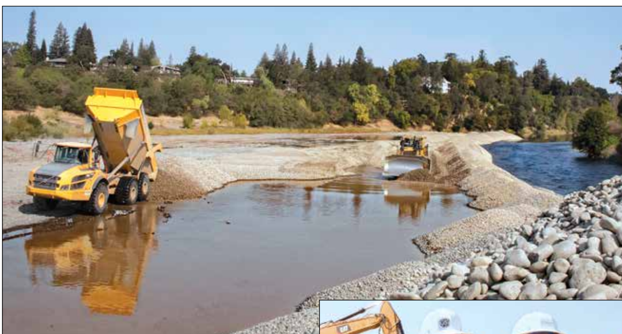
Above: Giant earthmovers relocate gravel in river shallows near Ancil Hoffman Park. The project will recreate natural spawning riffles for endangered migratory fish. Right: Water Forum Program Manager Erica Bishop (left) and communications officer Christine Kohn inspect habitat restoration sites in Carmichael reaches of the American River.
