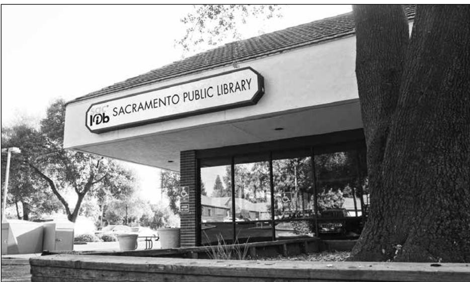
The Orangevale Public Library project doubled the building's footprint from 4,320 to 7,910 square feet, costing $950,000. Photo: Sacramento Public Library
