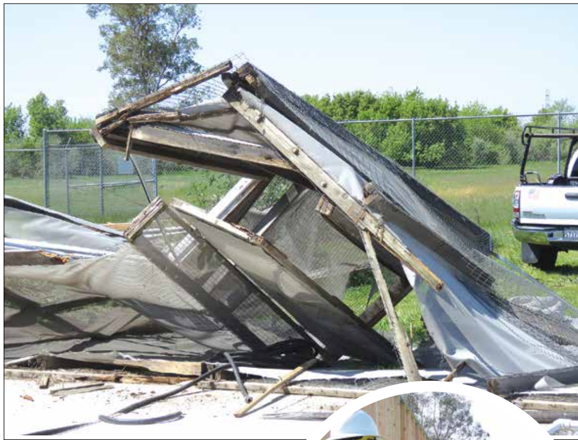
Above: February's gusty winds did some serious damage. Right: Volunteer workers employed by Wells Construction Corporation erect new walls for the Sacramento Wildlife Care Association's new aviary. Photos by Cecilia Lee Feser
