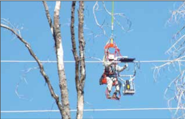
Suspended from a helicopter, a lineworker conducts X-ray photography on a SMUD transmission line in the Sierra. The work helps SMUD identify potential issues in advance so they can be repaired and help avoid power outages that could affect thousands of customers. Photo courtesy SMUD
