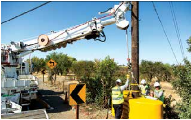
SMUD has seen an increase in “car-pole” accidents in recent years, so the electric utility is installing some measures to mitigate damage to power poles and other electrical equipment. The work is part of SMUD’s efforts to enhance public and worker safety and the SMUD grid’s reliability. Photo courtesy SMUD
