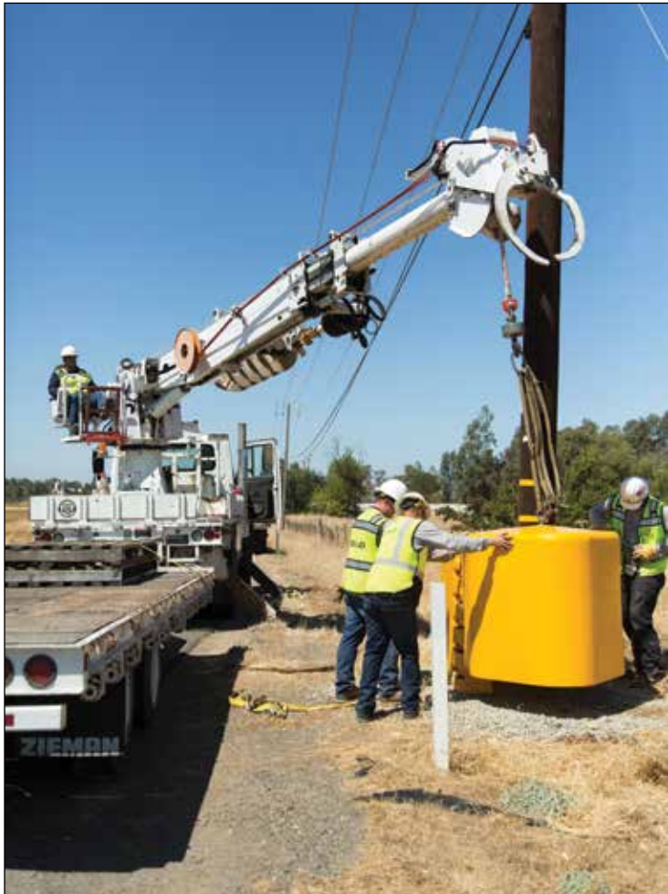
SMUD has installed some measures to mitigate damage to power poles and other electrical equipment by vehicles hitting them. The measures are part of a pilot program designed to increase visibility of and provide some protection to the power poles and to motorists. The work is part of SMUD's efforts to enhance public and worker safety and the SMUD grid's reliability. This photo shows a "Raptor" power pole barrier being installed in Wilton, CA. Photo courtesy SMUD
