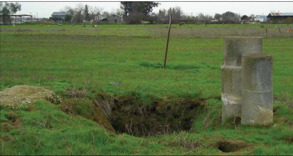
Children, animals, and even adults can fall into abandoned wells causing injury or death. Open pit wells and large-diameter drilled wells are particularly hazardous and often are hundreds of feet deep. Photo courtesy of Sacramento County.
